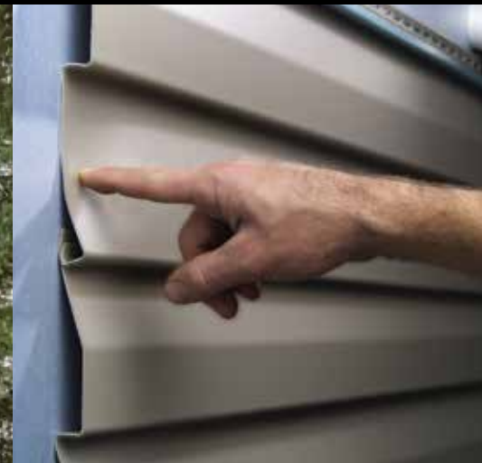
Traditional siding yields a hollow void between the siding and the wall.
